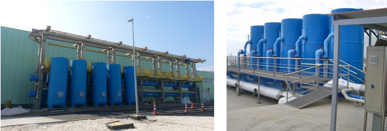
Fig. 1.2: Some aspects of different DrinTec™ contactors remineralization facilities.
