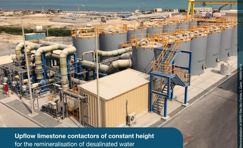
Upflow limestone contactors of constant height for the remineralisation of desalinated water
