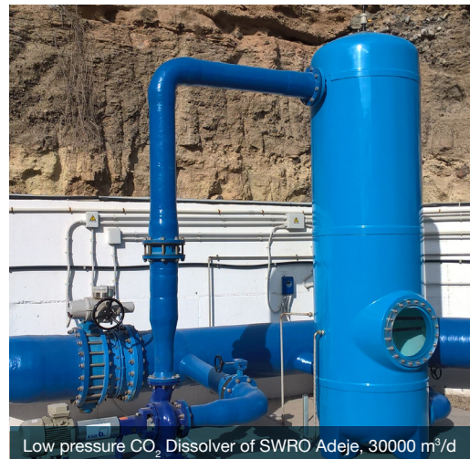
Low pressure CO 2 Dissolver of SWRO Adeje, 30000 m 3 /d
