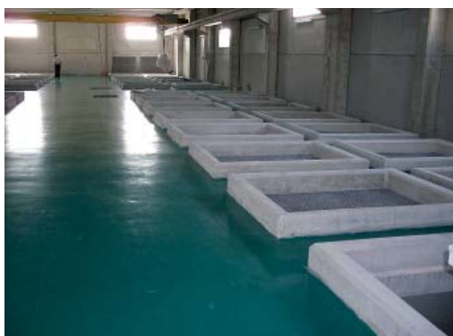
Figure 5.15: View of calcite silo charging area of an upflow constant height calcite plant
