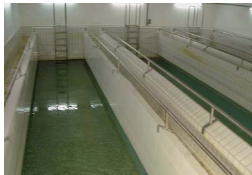
Figure 5.12: View of the cells of a downward flow calcite plant.
